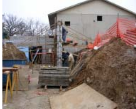
West to east view of loading dock wall-back of kitchen.
