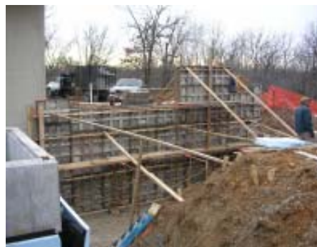
North to south view of loading dock wall on west side.
