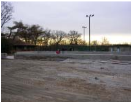
North to south view of new multi-purpose facility.
