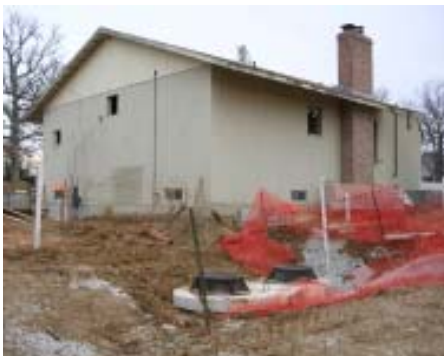
Southwest to northeast view of kitchen.
