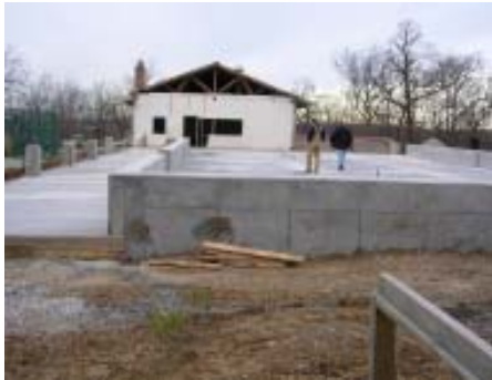
East to west view of the new multi-purpose facility foundation.
