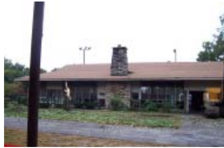
The last picture of the dining hall before the demolition began.
