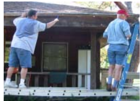
Mark Holmes and Past President Bob Weir remove gutters.
